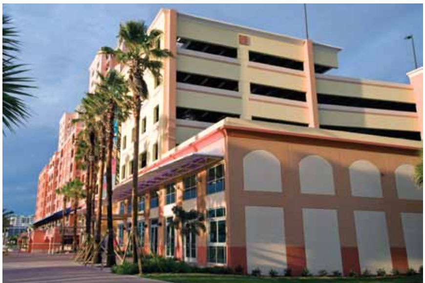
A speed ramp provides quick access to the first level of parking. It was placed above the first-floor restaurant space.
