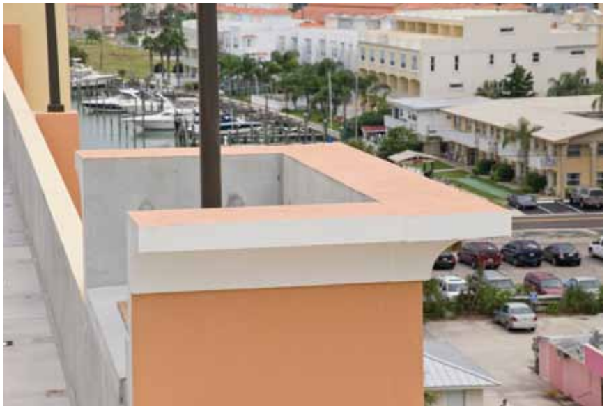
Improved durability and increased erection speed was achieved by integrally casting the cornice into the wall panels.
