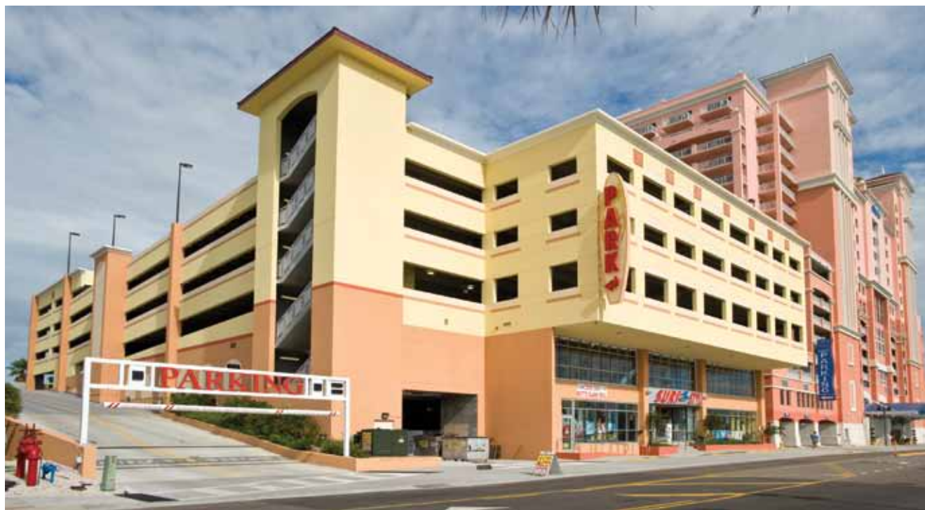
The Surf Style retail store and parking structure built along the beach in Clearwater, Fla., features a total-precast concrete structural solution that resolved a number of key challenges for the project while providing a strong aesthetic and fast erection.
