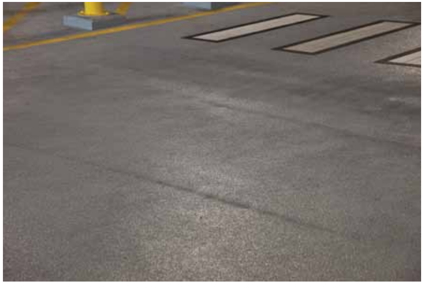
A Neoguard brand waterproofing was applied directly to the precast concrete double tees above the retail space to ensure a leak-free retail area below. Connections were cast for access from below as well to provide additional protection.
